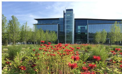
BANK OZK HEADQUARTERS LITTLE ROCK, ARKANSAS
